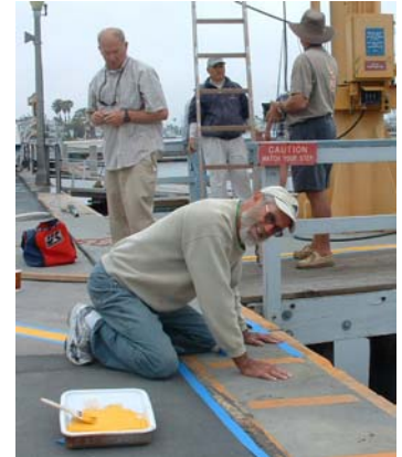
Dave Ellis painting the hoist area
